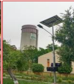
Solar Unit at Plant
