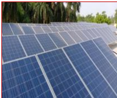
Roof of Central Canteen
