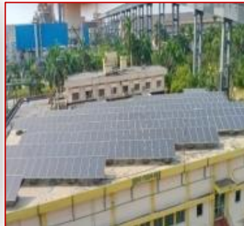
Roof of Urea-2 CR
